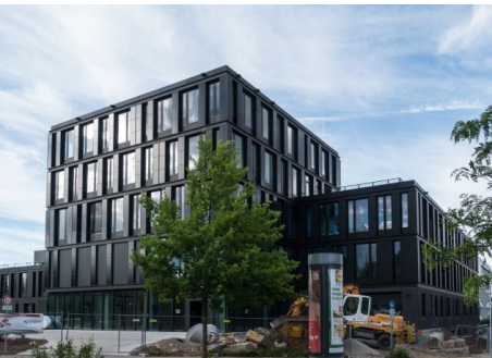
Stuttgart: Photovoltaics, Energy Policy and Energy Carriers, Central Division Finance, Human Resources & Legal
