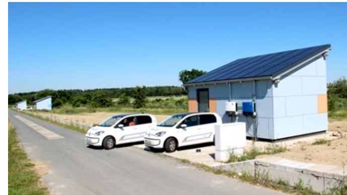
View of the experimental test setup in Fraunhofer IWES SysTec
