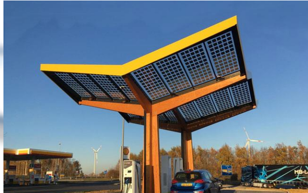
Source: Fastned fast charging station Uffenheim Germany (windkraft-journal.de)
