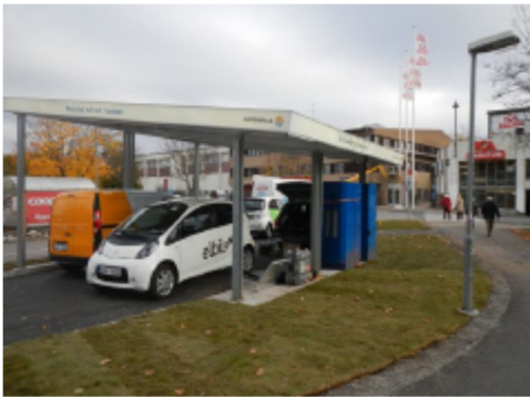
Figure 1. Fast charging station for electrical cars in Tyresö, Stockholm, Sweden.
